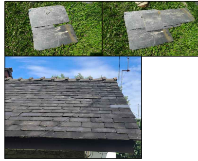
FIG.1.14: PICTURE OF EXISTING TILE AND TILE LAYOUT (AVG. L=1'-0"-1'-3", AVG. B= 0'-10"-1'-0") (NOT TO SCALE)
